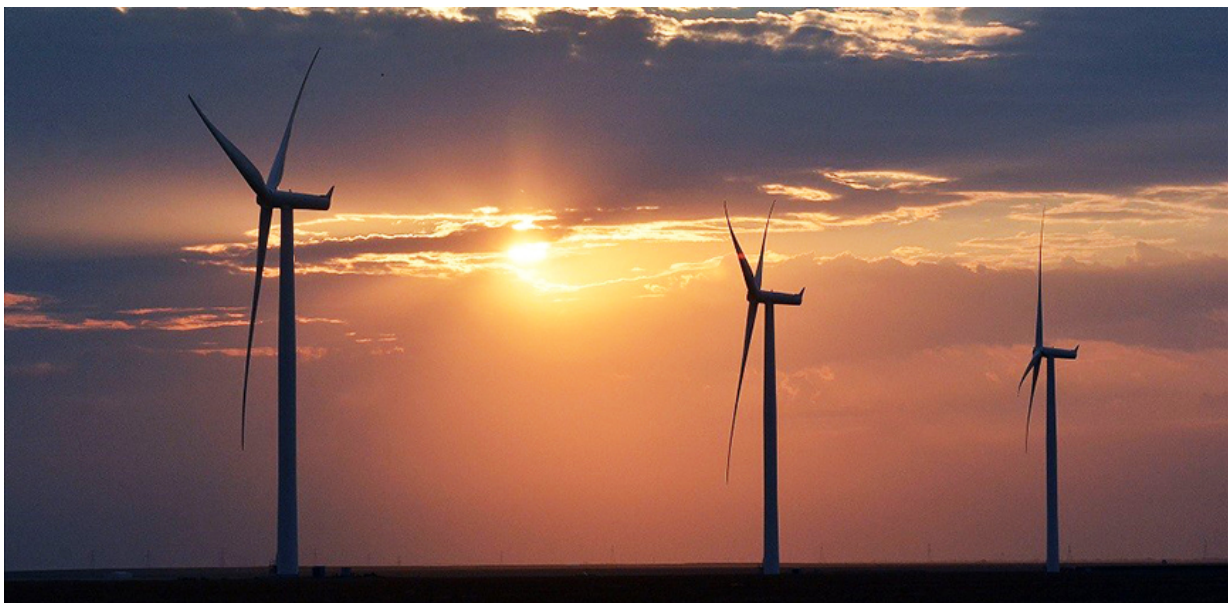
Pantex uses wind turbines to generate most of its energy.
